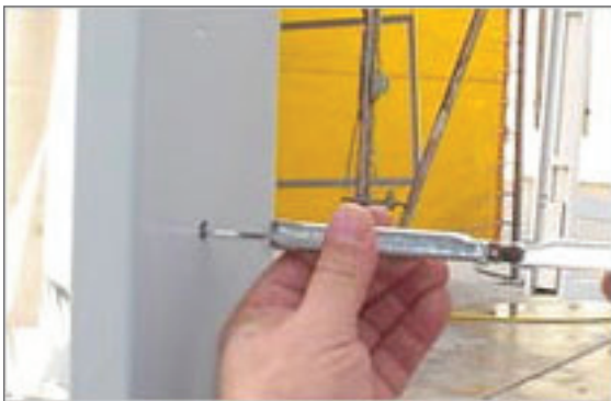
Adjust the pressure anchors.
