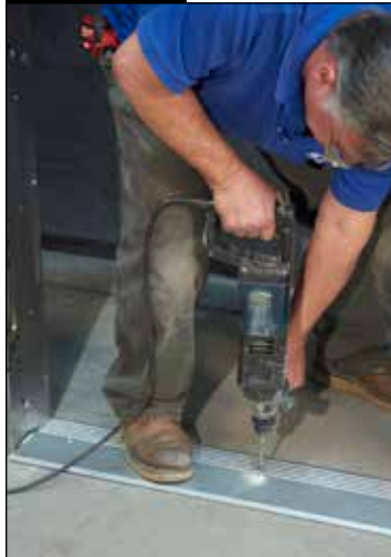
Drill thru threshold and install fasteners.
