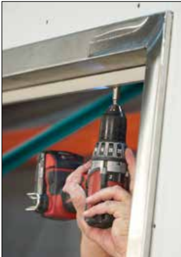
Install retainers notched end up. Install retainers with #10 hex head self-drilling screws and rectangular washers.
