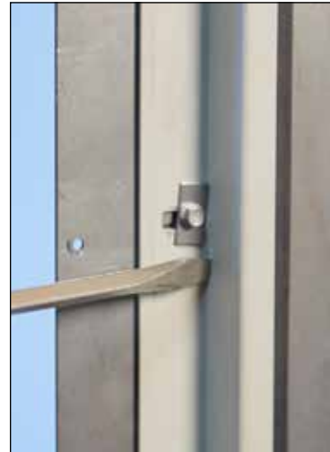
Washers should be installed parallel to retainers.
