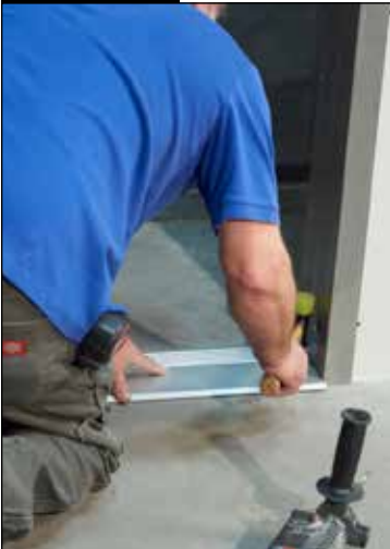
Install threshold over spreader.
