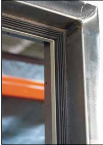
Install seals, glue corners with super glue or contact cement.
