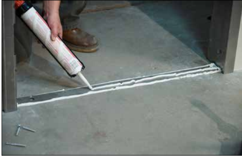
Caulk base frame spreader bar along sides and top.
