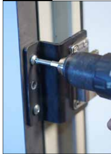
Install strike and begin seal adjustment. After seals are adjusted remove strike to install seal caps.
