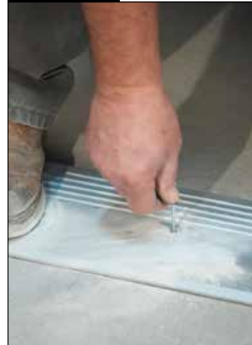
Install fasteners from top of threshold. Do not remove threshold for this step.
