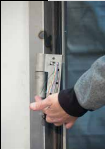
Install hinges on frame. Do not split hinges.
