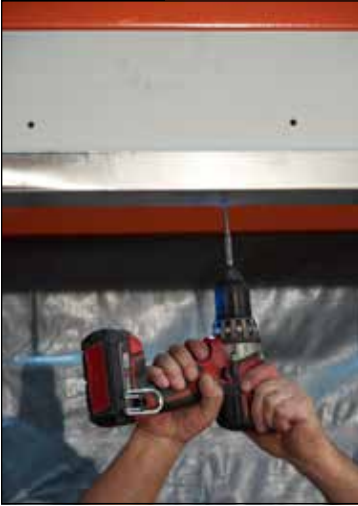
Secure trim frame to base frame with # 8 self-drilling screws.
