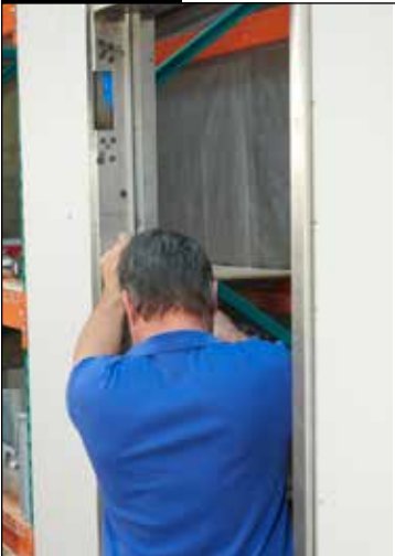
Install retainers notched end up. Install retainers with #10 hex head self-drilling screws and rectangular washers.
