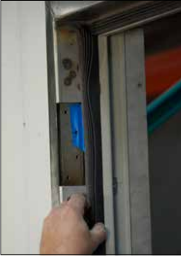
Install seals, glue corners with super glue or contact cement.
