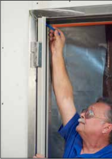
Measure retainers and cut to size. Do not cut notched ends.
