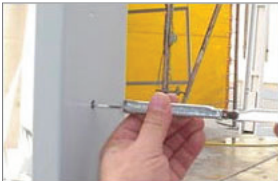
Adjust the pressure anchors.
