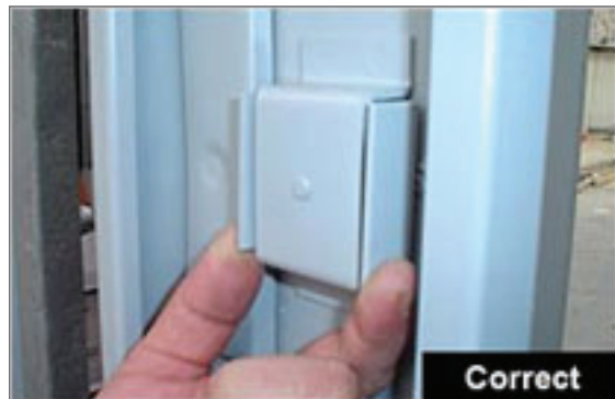
A properly adjusted pressure anchor is flush with the side of the frame.
