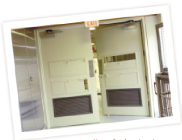
Above: Reinforced steel doors leading to the animal holding area.
